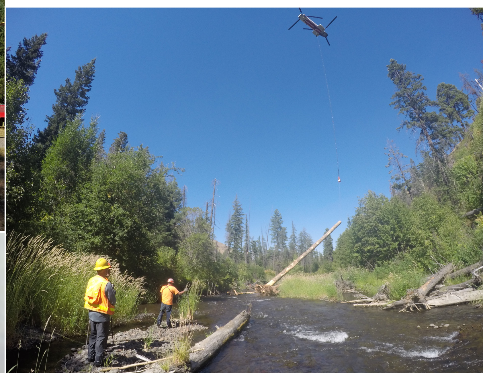
Helicopter crew placing large wood in the Tucannon River (July 2018)
